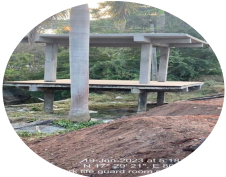
Life Guard Room under construction...
