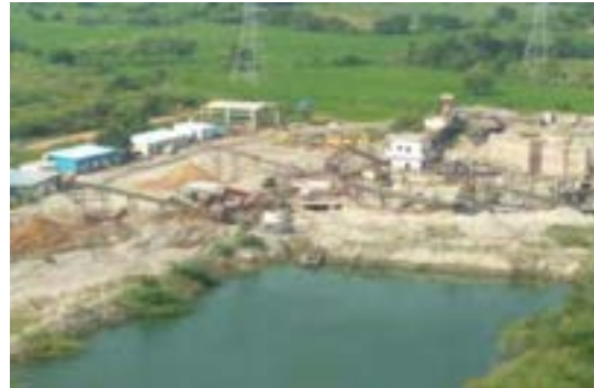
Processed Overburden Plant at Ramagundam-MOCP (15 LCM/annum)
