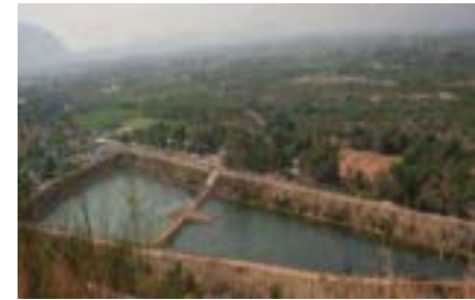
Creation of Summer Storage Tank
